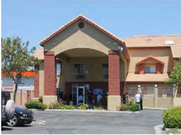
A former motel in Fontana has been converted into the Path, a Homeless Prevention Resource and Care Center located at 17133 Valley Boulevard. Officials gathered for a ribbon-cutting ceremony on July 1.
